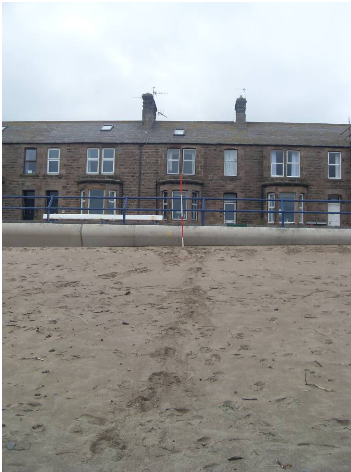
Plate 4 – Survey photograph 1aBTBC11_20111013_Up.JPG
